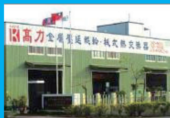
· Kaohsiung Taiwan Plant
